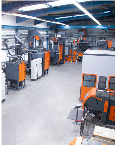
CEC Shot Blasting
